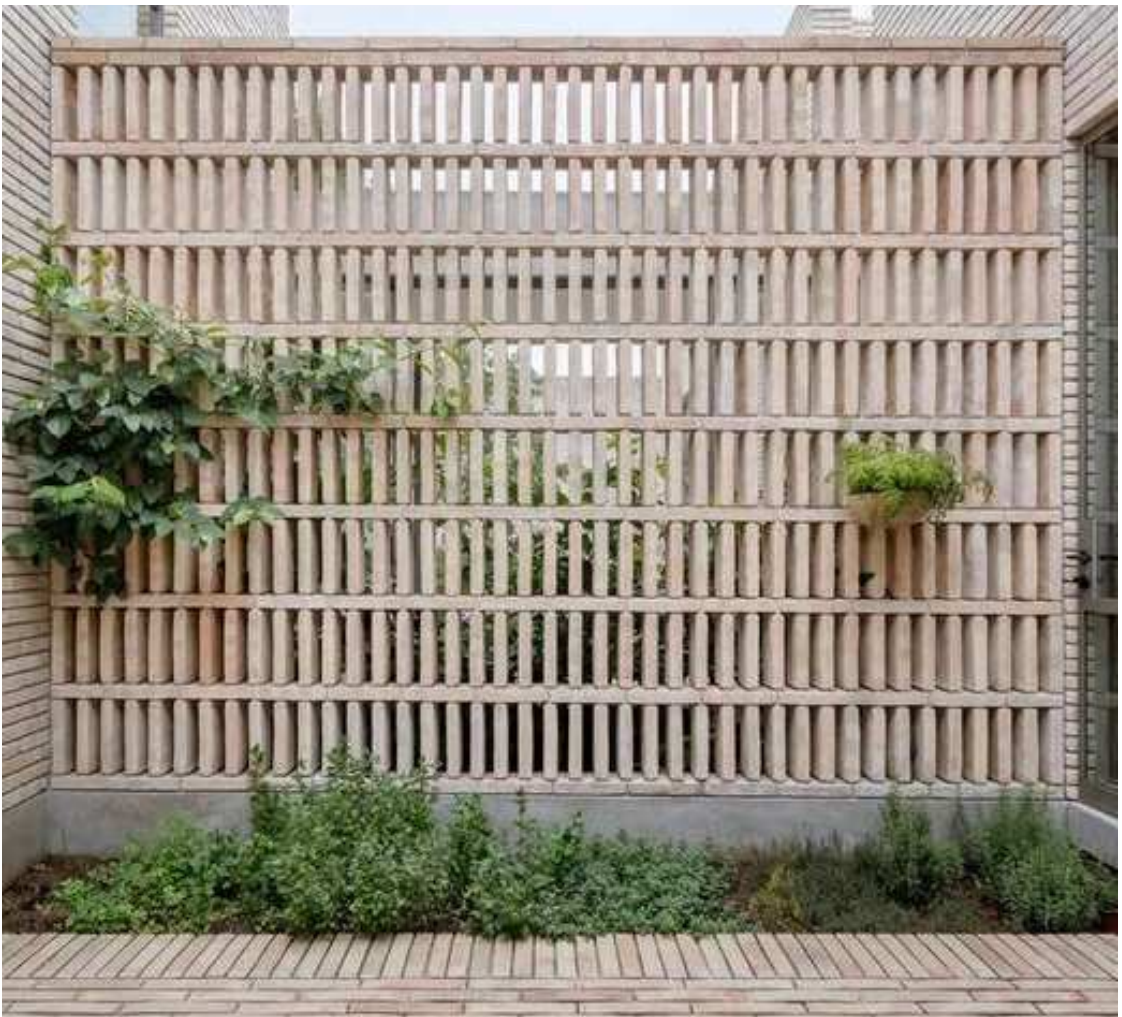
PROPOSED DETAIL OF MASONRY BREEZEBLOCK WALL
