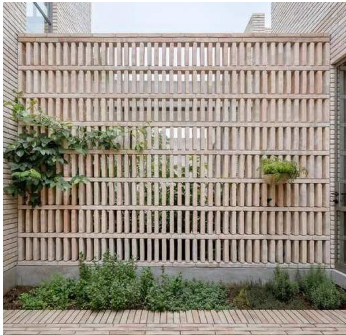
PROPOSED DETAIL OF MASONRY BREEZEBLOCK WALL
